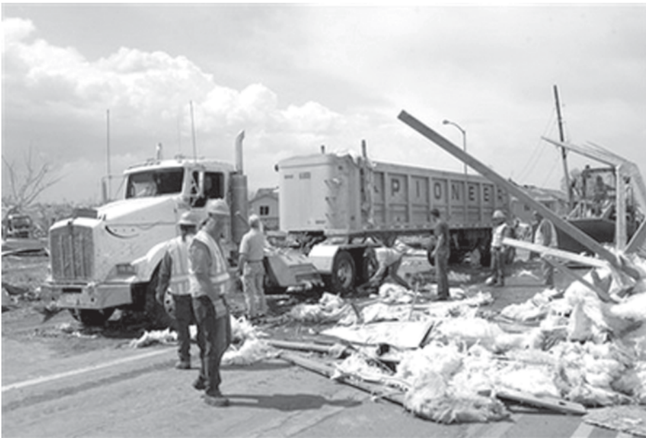
Colorado Dept of Transportation workers remove debris from a truck that was hit by the roof of a nearby building when a tornado touched down, on 22 May, 2008 in Windsor, Colo. A large tornado tore through several northern Colorado towns on Thursday, killing at least one person and flipping over tractor-trailers, toppling freight rail cars and ripping roofs off buildings.
