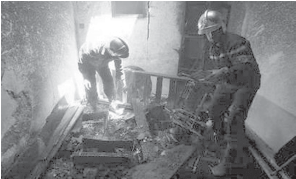
Firemen inspect a burnt house in Berriane, 40 km (25 miles) north of Ghardaia, on 18 May, 2008. Hundreds of Algerian security forces were deployed in the town of Berriane on Sunday to try to end three nights of clashes between Arabs and minority Berbers, the worst urban unrest in the OPEC producer in months.—INTERNET
