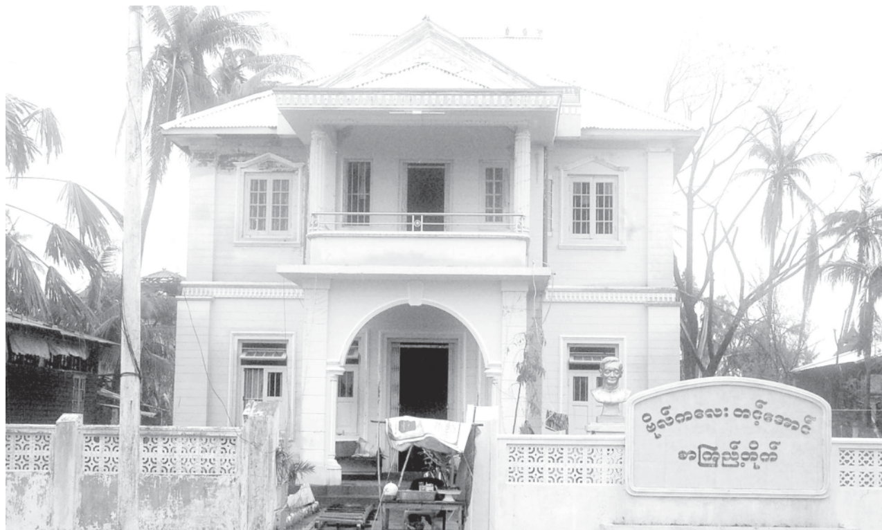
A library seen after being repaired in Bogale.—MNA
