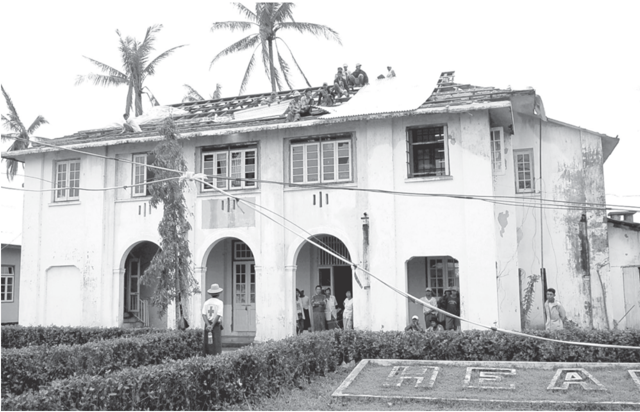
Labutta Township People's Hospital under repair.
