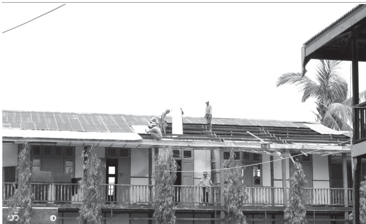
Basic Education High School of Mawlamyinegyun Township under reconstruction.—MNA
