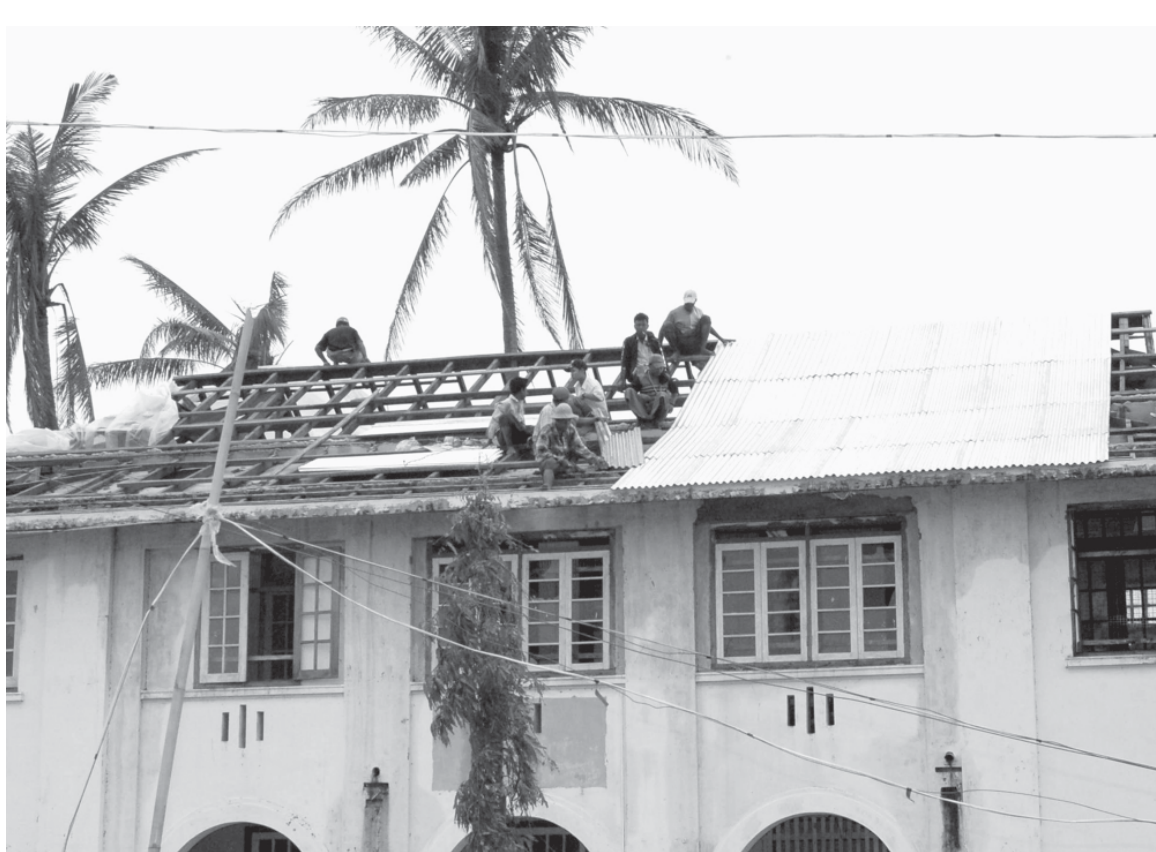
Labutta People's Hospital under reconstruction.—MNA
