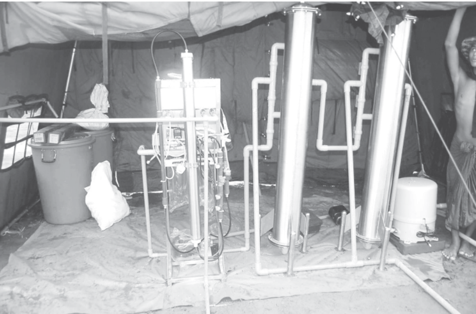
Water purifiers donated by foreign countries being installed at Kyonda Village. — MNA
