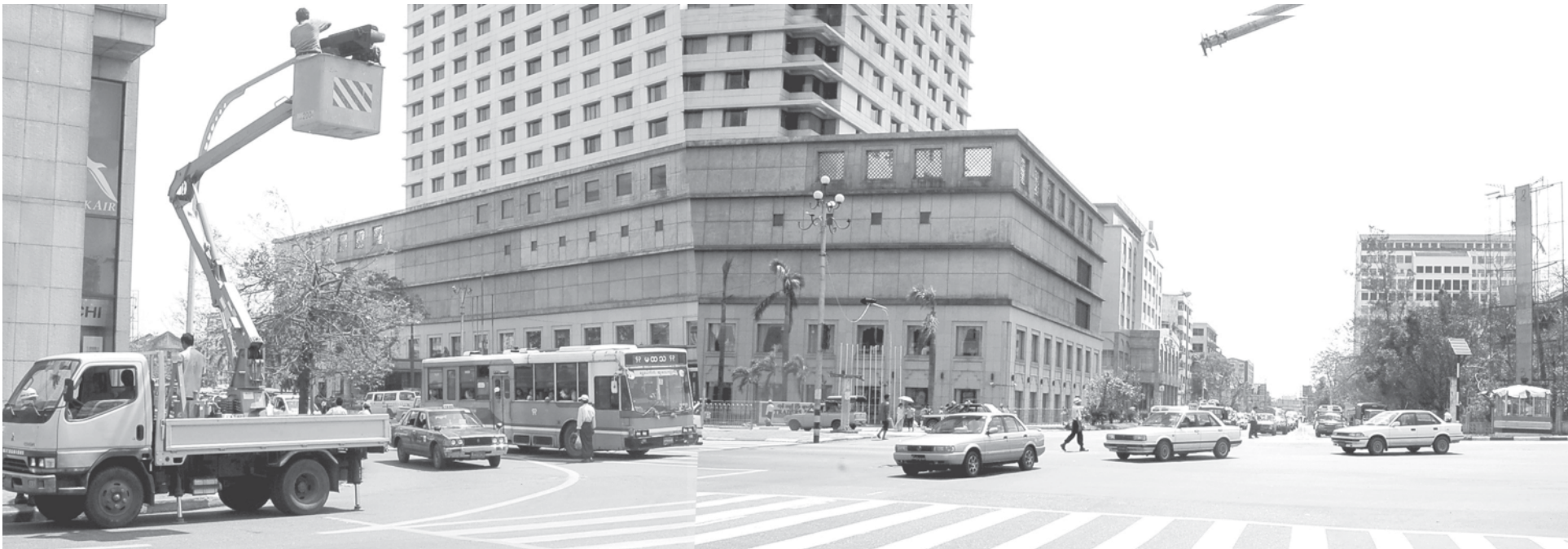
Traffic lights being repaired on Sule Pagoda and Bogyoke Aung San Streets in Yangon.—MNA
