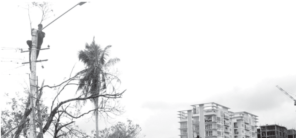
Service personnel of Hline electric engineer's office install power lines for resuming power. —MNA
