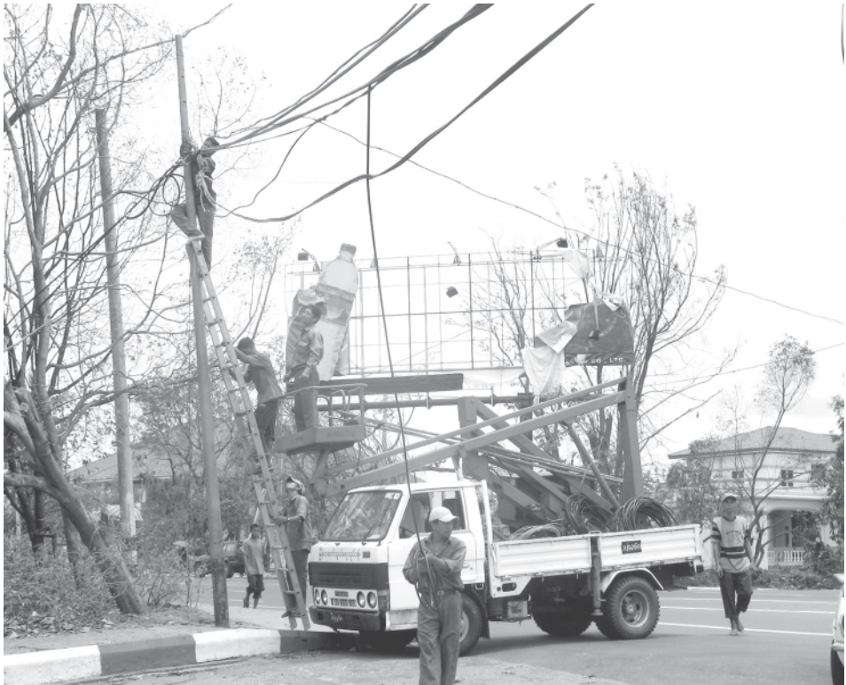
CPT employees repairing telephone lines in Yangon.—MNA
