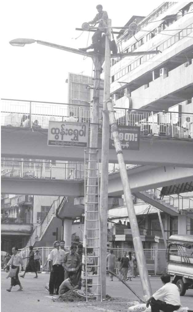
Staff of Myanma Electric Power Enterprise repair a damaged lamp post caused by storm on Maha Bandoolla Street.—MNA
