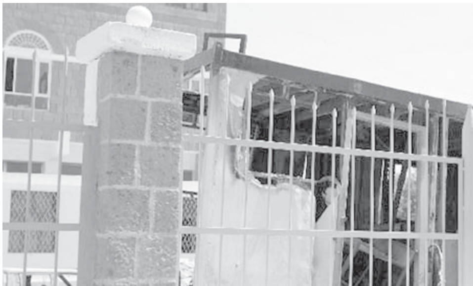
Damaged property is seen at the parking lot of the Customs authority in Sanaa on 30 April, 2008. Unidentified attackers fired two shells at the government office near the Italian Embassy in the Yemeni capital Sanaa early Wednesday, but there were no casualties, a security source said.—XINHUA
