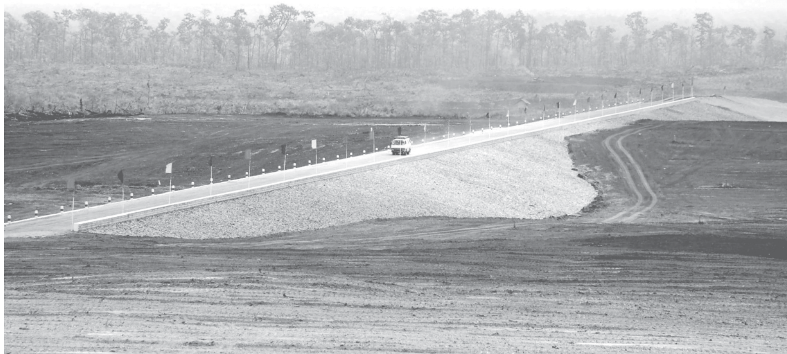
Kyaingkhram Dam under construction in Yaksawk Township.—MNA
