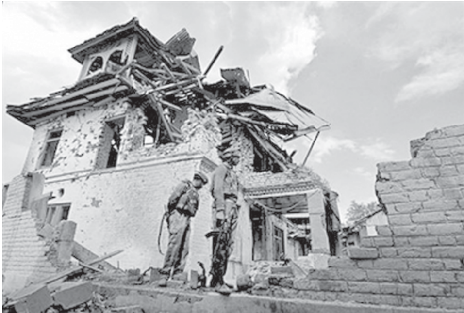
Indian soldiers inspect the damage to a house after a firefight in Baramullah, some 58kms north-west of Srinagar.—INTERNET
