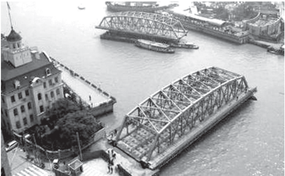
A general view of the Waibaidu Bridge, which has been dismantled into two parts, at the Bund in Shanghai on 6 April, 2008. Shanghai's oldest bridge across the Suzhou River, the Waibaidu Bridge, which has a history of at least a century, is dismantled and taken to dry docks for refurbishing and will be reset after nine months repair, local media reported.—INTERNET
