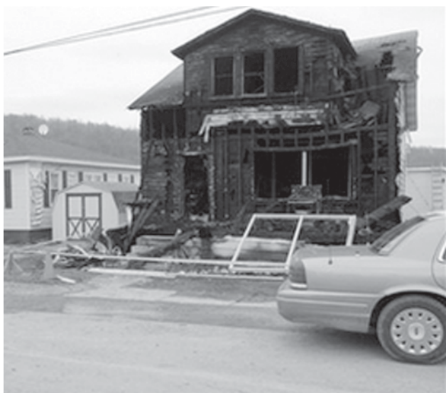
Photo shows the house where ten people died in a house fire on 3 April, 2008. Officials have said ten bodies have been recovered, while two others survived, according to the state police.—INTERNET
