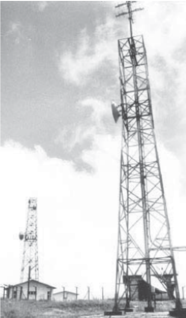
A microwave station seen in Haka Township of Chin State.
