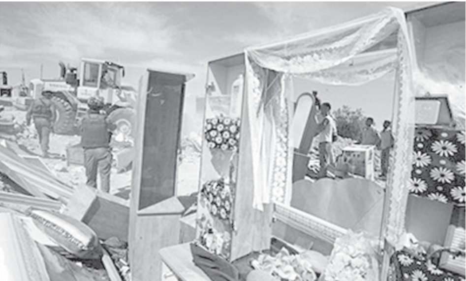
Belongings of a Palestinian family are seen outside their house as an Israeli army bulldozer demolishes it, south of the West Bank town of Hebron on 19 March, 2008. The house was built without construction permission. —INTERNET
