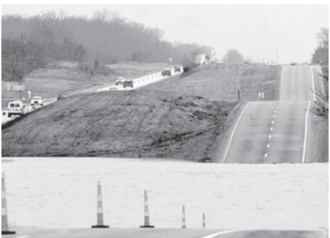
Traffic is diverted (L) along US Highway 60 after floodwaters spilled over a section of the roadway east of Springfield, Missouri, on 21 March, 2008. —INTERNET
