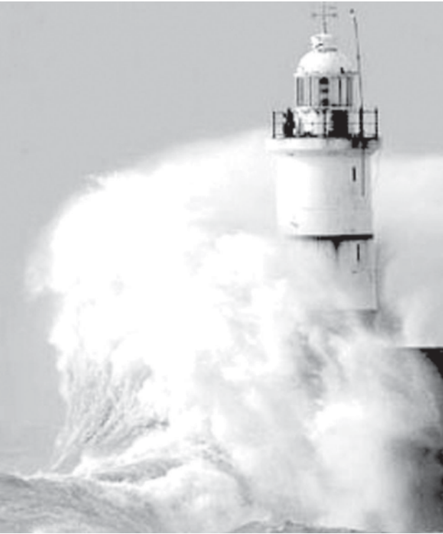
Stormy seas hit coastal sea defences and a lighthouse at Seaford in Sussex in southern England on 10 March, 2008. A storm rushing in from the Atlantic lashed the south west on Monday as high winds and tides brought the risk of coastal flooding.
