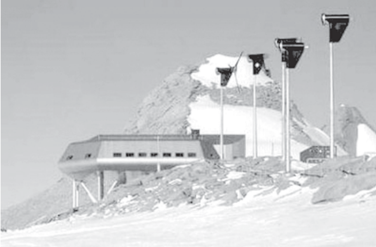
View of the Belgium’s Princess Elisabeth polar station, received at a news conference on the first phase its construction, in Brussels March 11, 2008. Belgium is building the first ever zero-emission polar station in the Antarctic, powered by solar panels and wind turbines and designed to have minimal impact on the climate change its scientists are studying. —INTERNET
