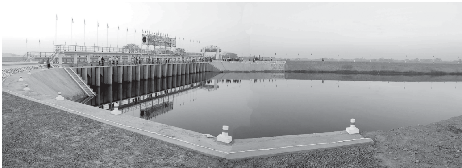
Takaw Sluice Gate in Thongwa Township. — MNA
