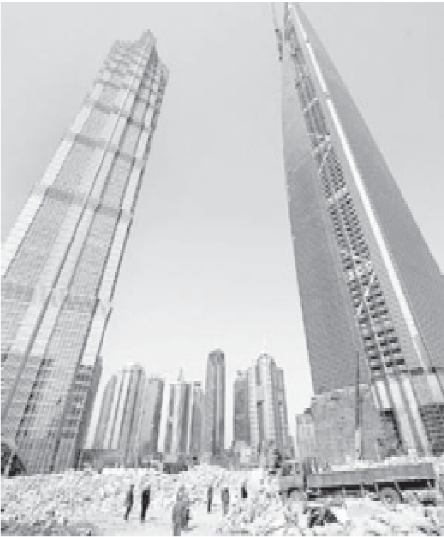
Workers level ground at the construction site for Shanghai Centre, the city's planned new skyscraper. Located in Lujiazui, Pudong, the building is expected to soar to 580 metres, dwarfing the 421-metre Jin Mao Tower and the 492-metre Shanghai World Financial Centre in its neighbourhood.
