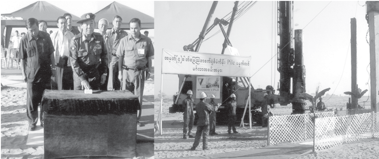
Minister Brig-Gen Lun Thi presses a button to launch work on construction of No 4 Fertilizer Plant in Hmawby Township. — ENERGY
