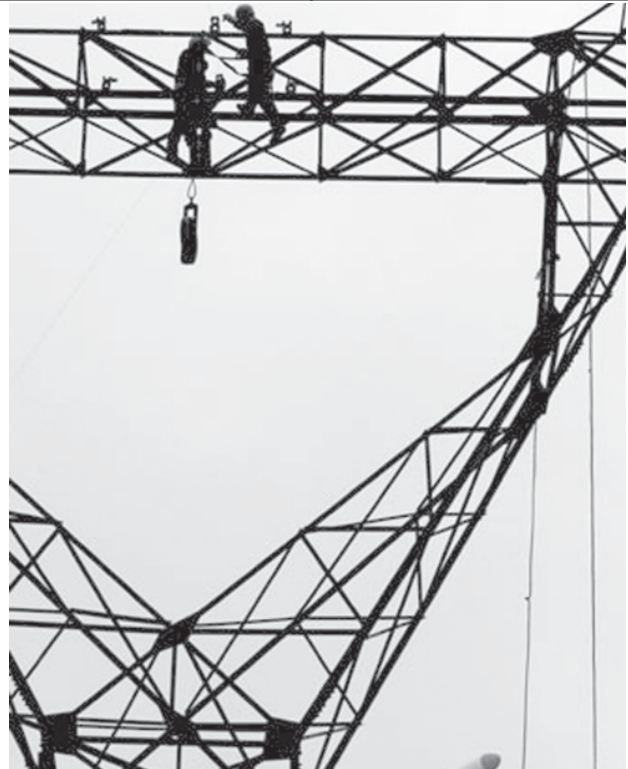
Workers repair a power line on a steel tower with the help of a line-laying airship, in Guiyang, capital of southwest China's Guizhou Province, on 17 Feb, 2008.— INTERNET
