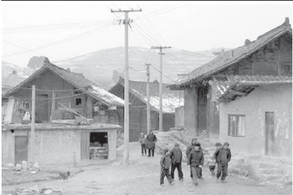
Residents walk past power poles, damaged by snow, in Guizhou Province. Transport, power generation and food supply were back to normal in most of China on Sunday.
