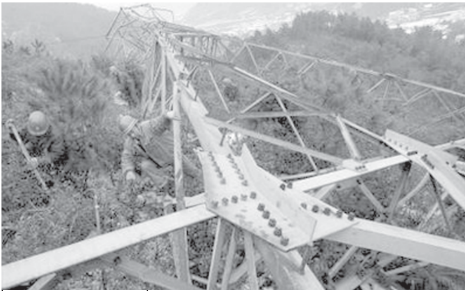
Workers check a power supply tower which had collapsed during heavy snowfall in Wuhan, Hubei Province, on 5 Feb, 2008.
