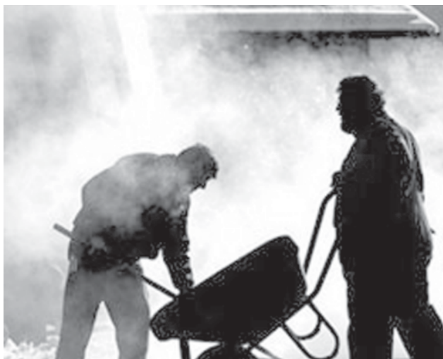
Men work at a construction site in Germany.
