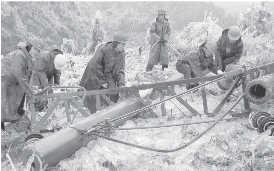
Employee of local power supply bureau repair electricity transmission line in Zhaoping County, south China's Guangxi Zhuang Autonomous Region, on 1 Feb, 2008. Over 300 employees of local power supply bureau were called on to repair electricity transmission line damage caused by continuous heavy snow and frost to ensure safe power supply in the county. —XINHUA
