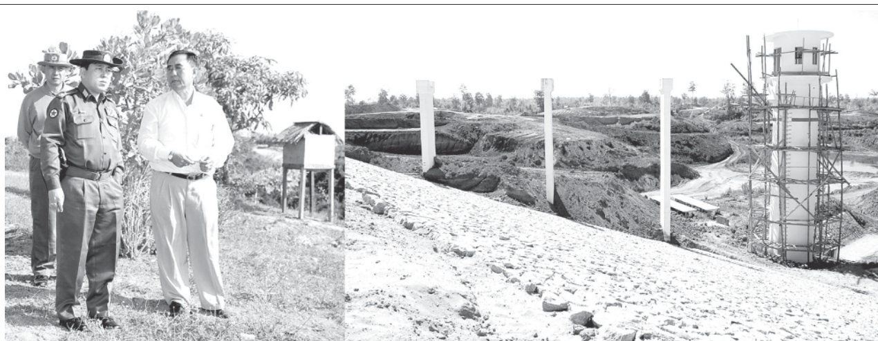
Commander Maj-Gen Wai Lwin inspects construction of Madan Dam Project in Nay Pyi Taw Lewe Township. — MNA
