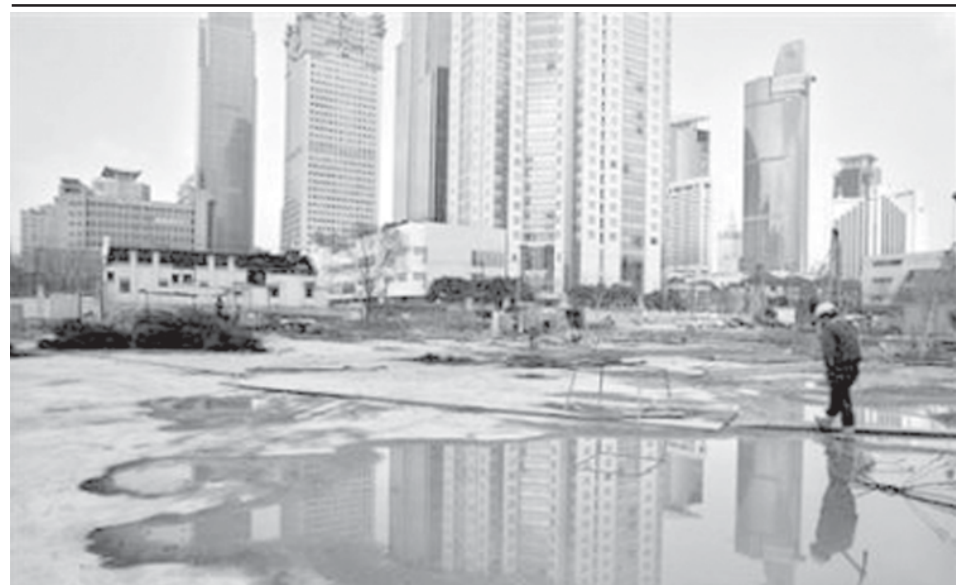
A worker walks in a new five-star hotel construction site in downtown Shanghai, on 24 Jan, 2008. China's economy grew 11.4 percent in 2007, the fastest pace in 13 years.—INTERNET
