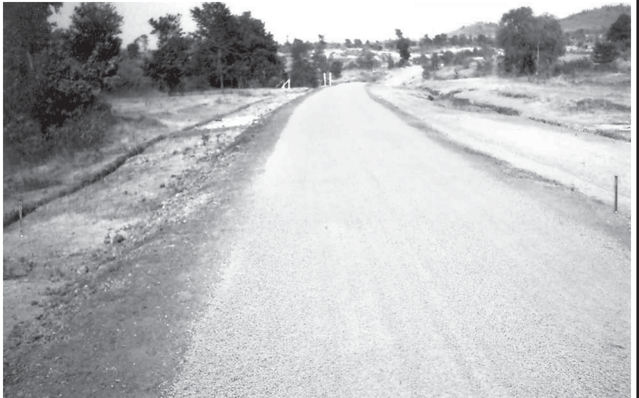
The road section in Natmauk Township has been upgraded to a tarred facility.
