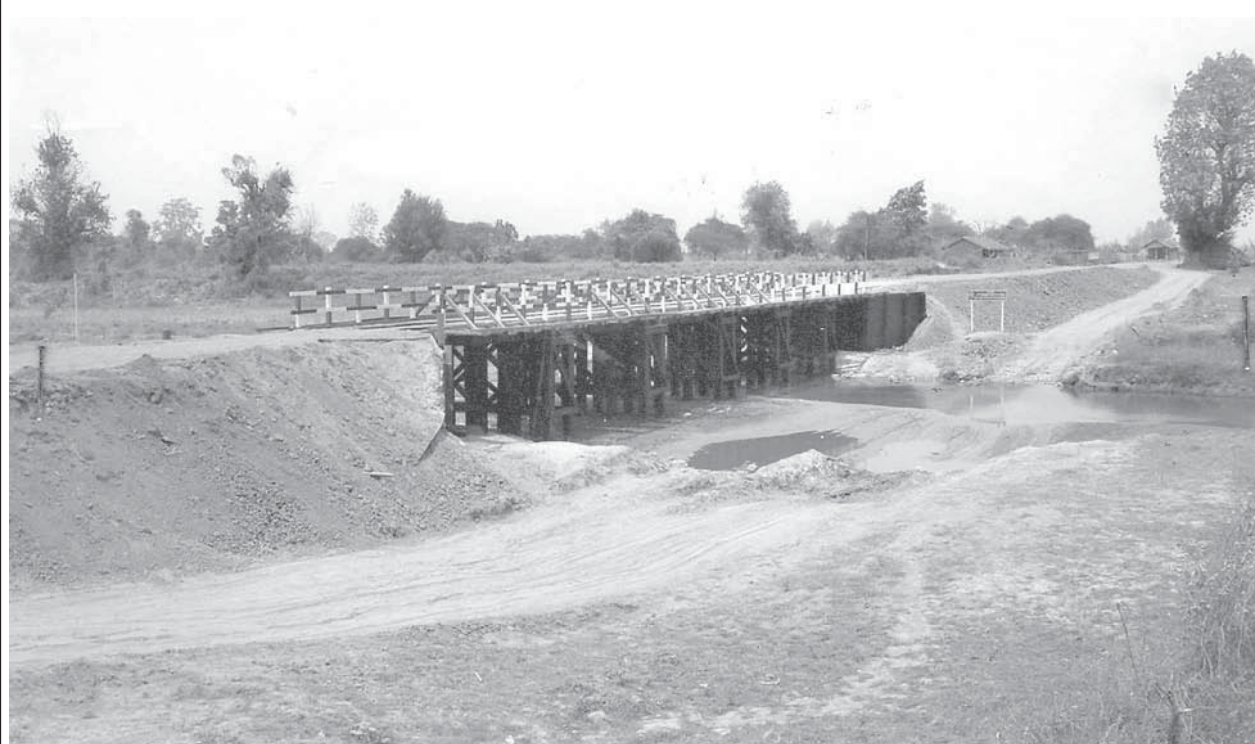
A 120' x 14' wooden bridge on Nyaung Creek near Yaypyae Village in Taungdwingyi Township.
