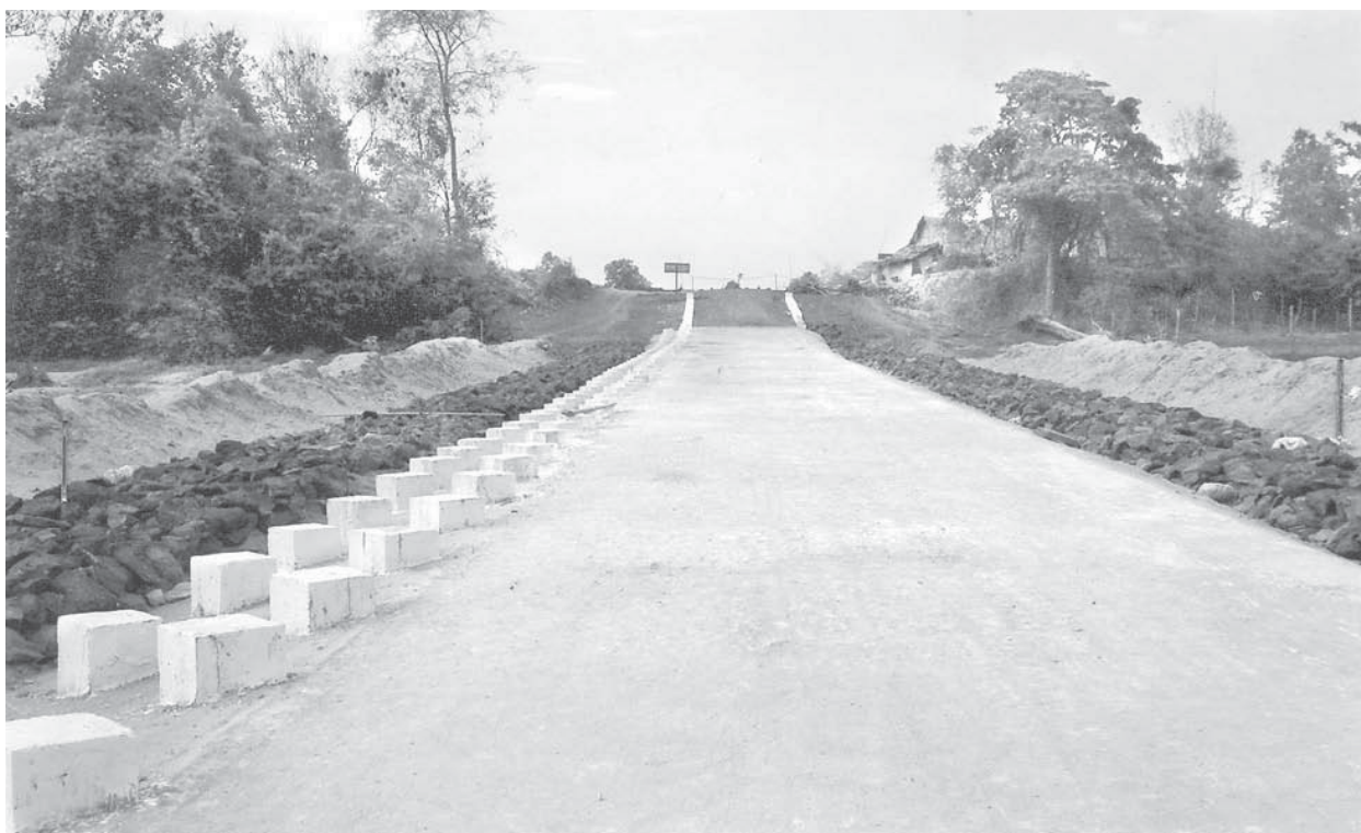
A 700' x 18' Phayonchaung Bridge near Konbo Village in Hsinbaungwe Township.
