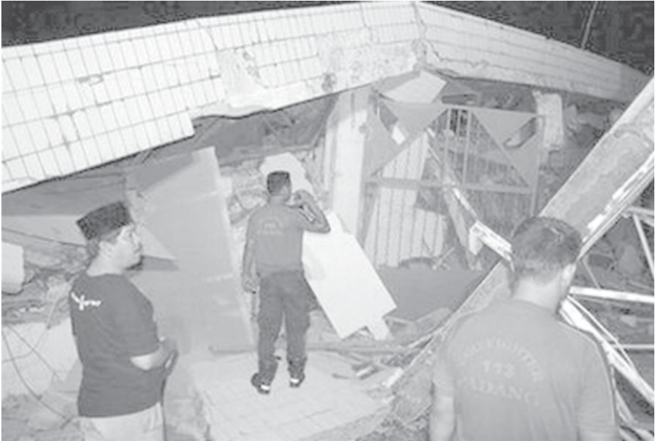
A resident and firefighters look at a damaged building after a strong earthquake struck in Padang, Indonesia’s West Sumatra Province on 12 Sept, 2007. —INTERNET
