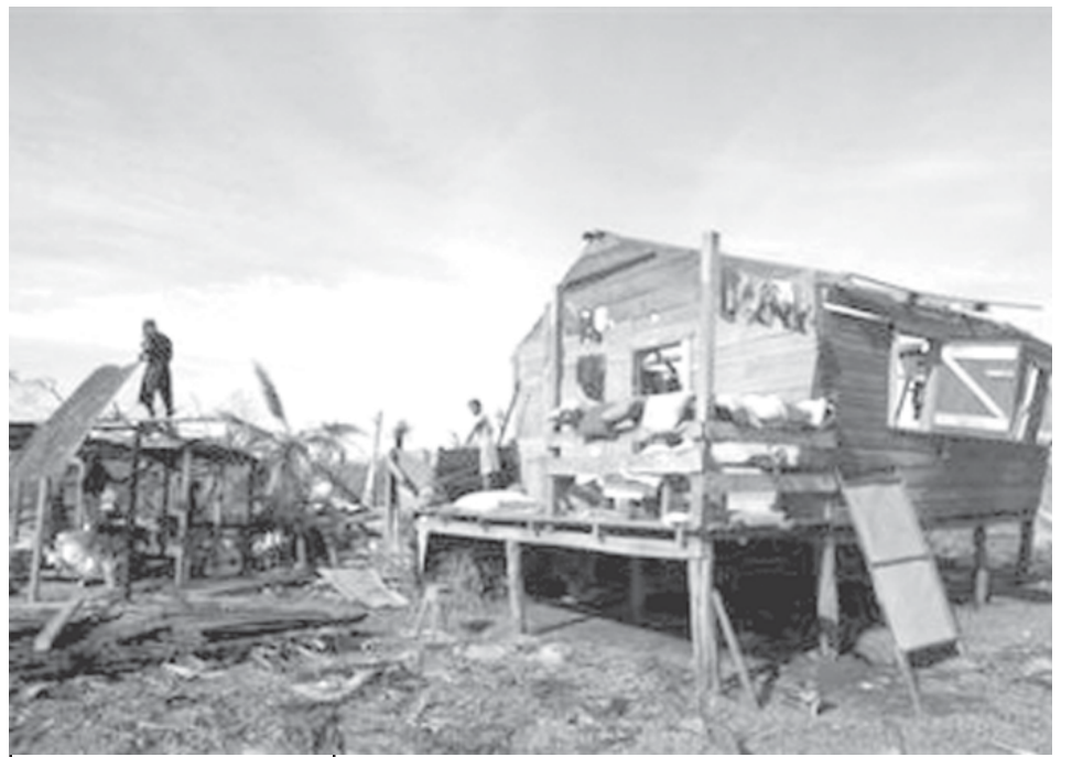
A Miskito Indian man repairs his house, damaged by Hurricane Felix, in the small town of Krukira on the Caribbean coast of Nicaragua on 6 Sept, 2007. — INTERNET
