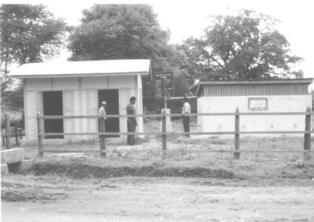
Officials of Taze Township Development Affairs Committee inspected a tube-well in Zipauk Village, Taze, Sagaing Division recently. A 10-year plan is being implemented to supply drinking water to rural areas in Sagaing Division. — H
