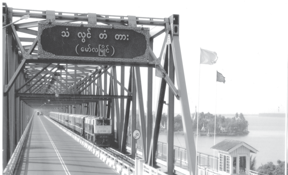
Thanlwin Bridge across Thanlwin River in Mawlamyine.
