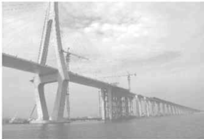
Photo taken on 21 June, 2006 shows the bridge under construction spanning Zhanjiang Gulf in Zhanjiang, south China's Guangdong Province. The two sections of the main bridge were joined on the morning of Wednesday. The length of the bridge is 3,981 metres and its main tower is 155.11 metres high.—INTERNET
