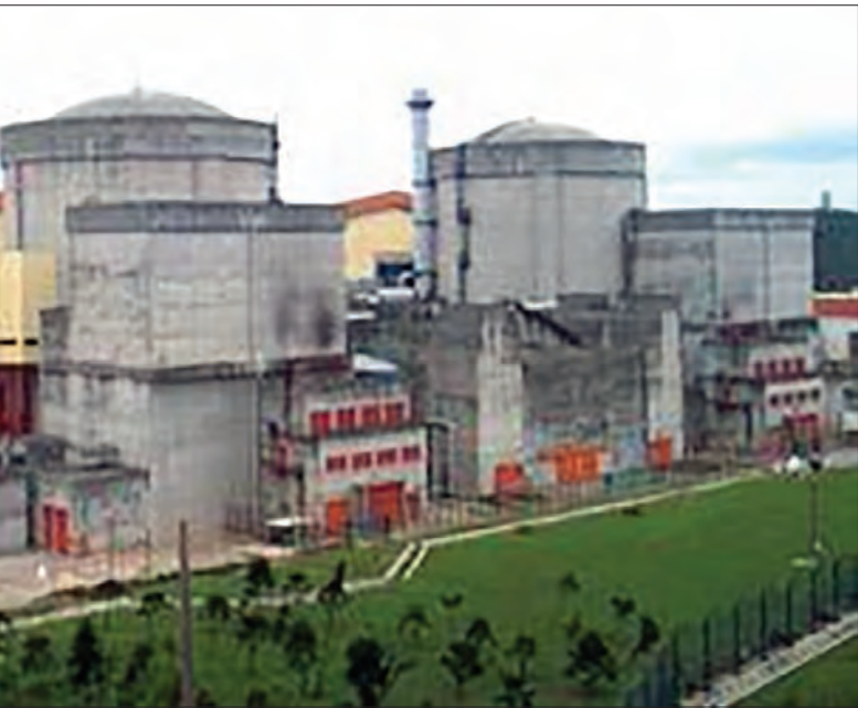
Station. PHOTO: COURTESY OF CLP POWER
