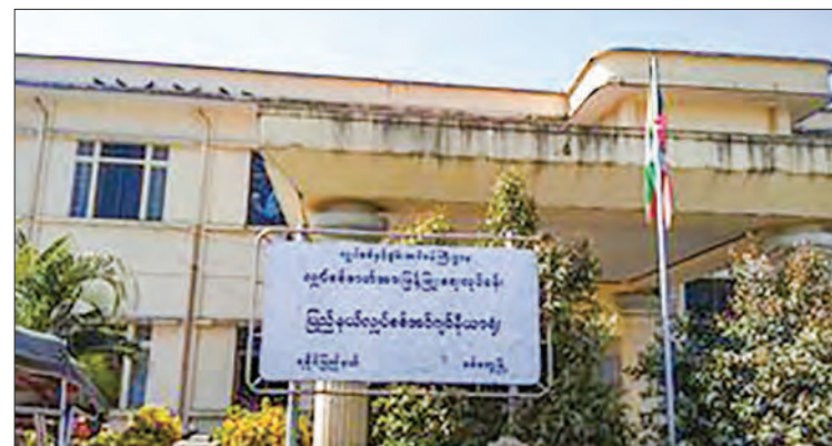
Rakhine State Electric Power Enterprise has arranged to prevent outage during the examination period. PHOTO: TIN TUN (IPRD)
