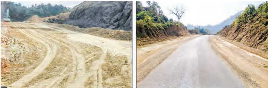
12ft wide bituminous road construction between 12.8km and 13.2km at Buthidaung-Maungdaw road
