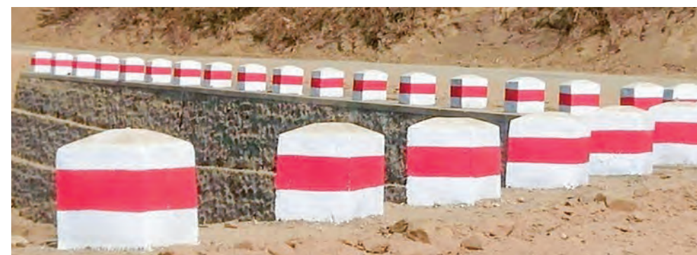
Completion of retaining wall
