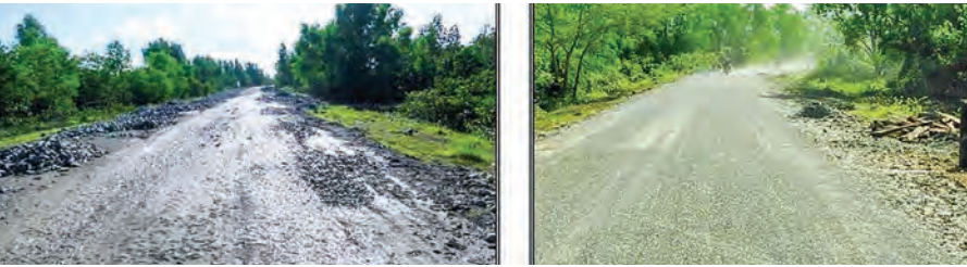
Before construction at mile post (68/0-68/5)
