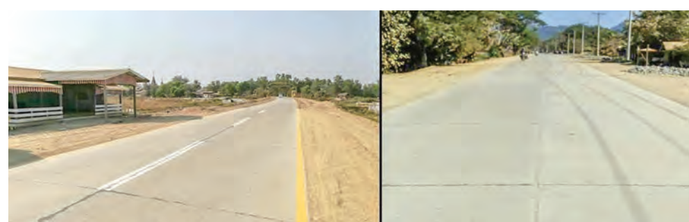
Completion of concrete road
