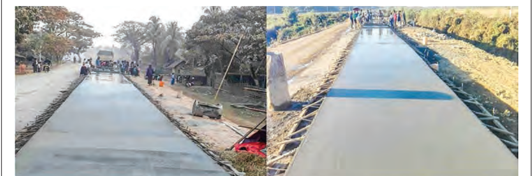
Ongoing construction of concrete road
