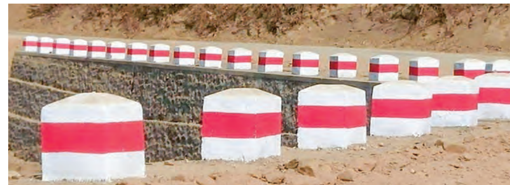
Completion of retaining wall
