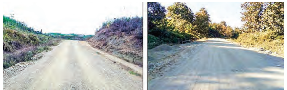
After construction of bituminous road between (53.2km-53.4km)
