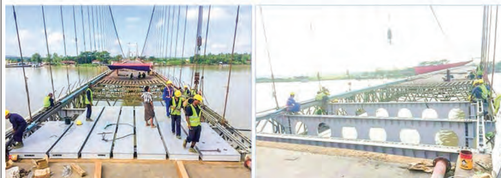
Rehabilitation of Ramong suspension bridge on Yangon-Sittwe road
