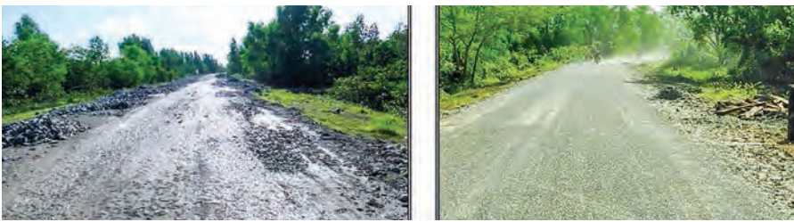
Before construction at mile post (68/0-68/5)
