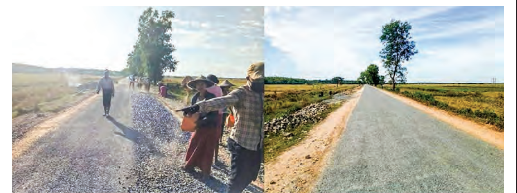
Construction of 0.8m wide bituminous pavement (160.6km to 161.4km) on Yangon-Sittwe road
