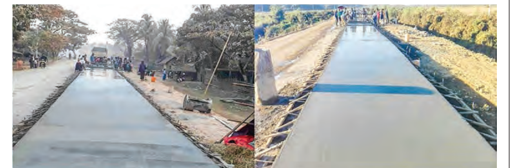
Ongoing construction of concrete road
