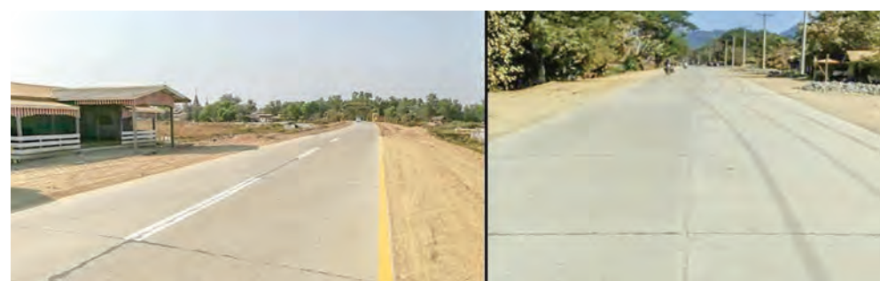
Completion of concrete road
