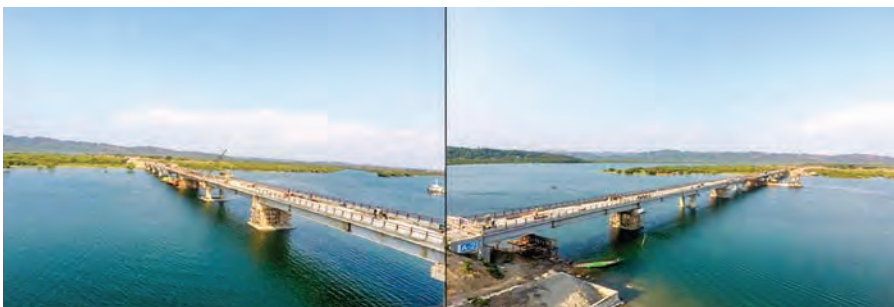
365.7m length reinforce concrete bridge construction (Tawphyar bridge) at Ponnagyun- Rathedaung road
