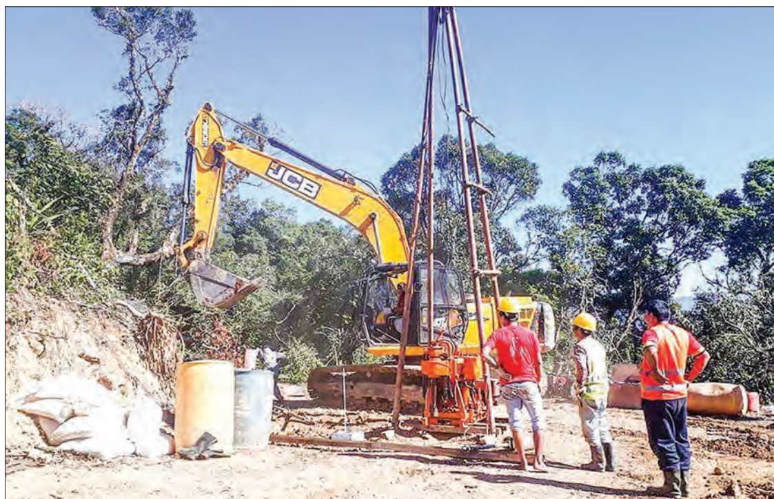
Engineers carry out geotechnical investigation to construct small airport in Lailenpi. PHOTO: SUPPLIED
