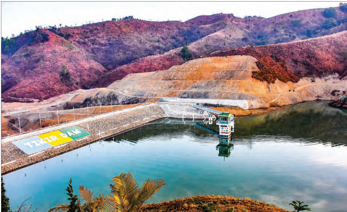
Tikir Dam will irrigate highland farms and produce 50 kilowatts of electricity through a mini-hydroelectric power station. PHOTO: MNA
