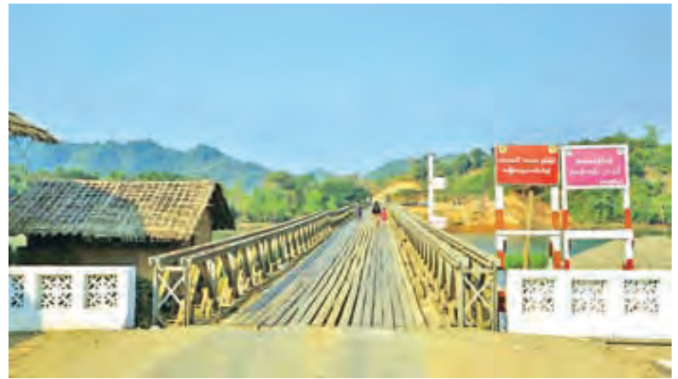
Darlet Chaung Bridge on the Minbu-An-Sittway road.
