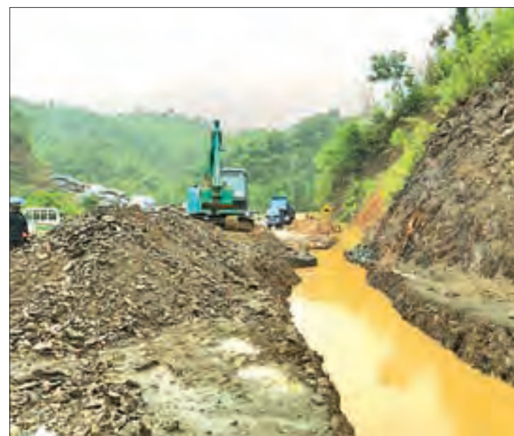
Backhoes are used to fill in parts of the Sittway-Yangon highway that have eroded due to flooding from heavy rains. PHOTO: YE HTUT
