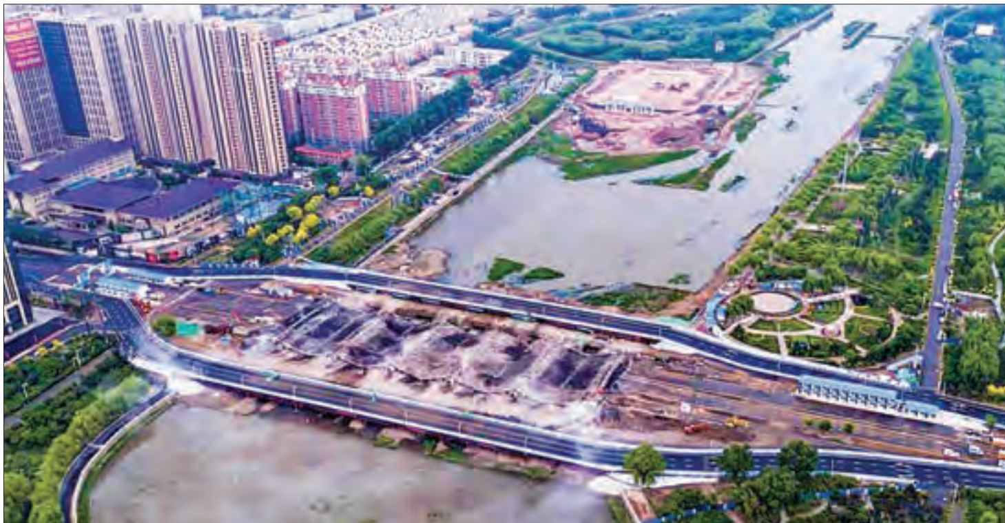
The Changchun Ziyou Bridge is seen after a controlled explosion in Changchun, capital of northeast China's Jilin Province on 31 May, 2017. Based on investigation and calculation, the explosion was designed to demolish only the deck of the bridge. Its pillars were preserved. After the explosion, a new bridge will be built in the next 5 months. PHOTO: XINHUA
