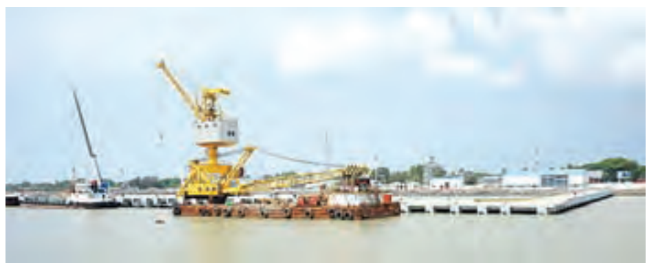
The dredging sand banks.
