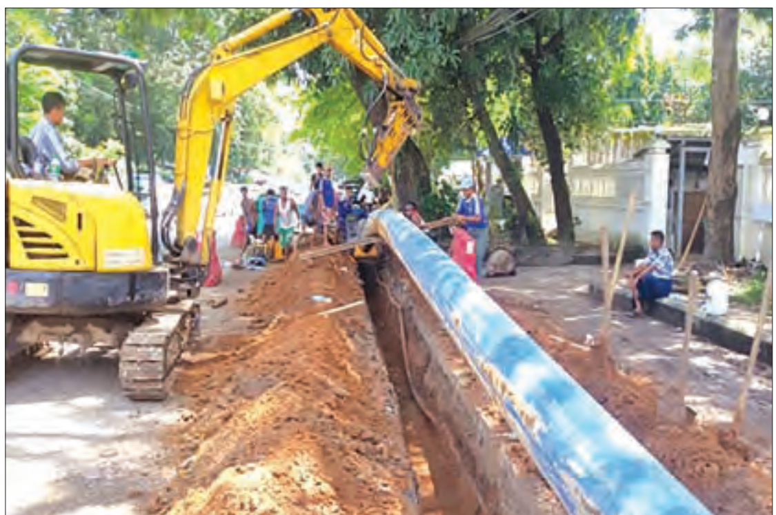
Laying of underground water pipelines in Yangon. PHOTO: MNA
