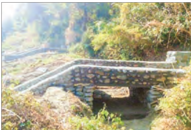
Canal bridges in Thinchau Village in Mindat Township. PHOTO: MNA
