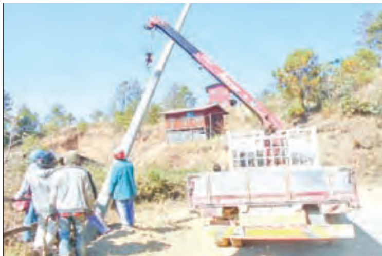
A concrete post for the 11Kv powerline in Haka erected. PHOTO: MNA
