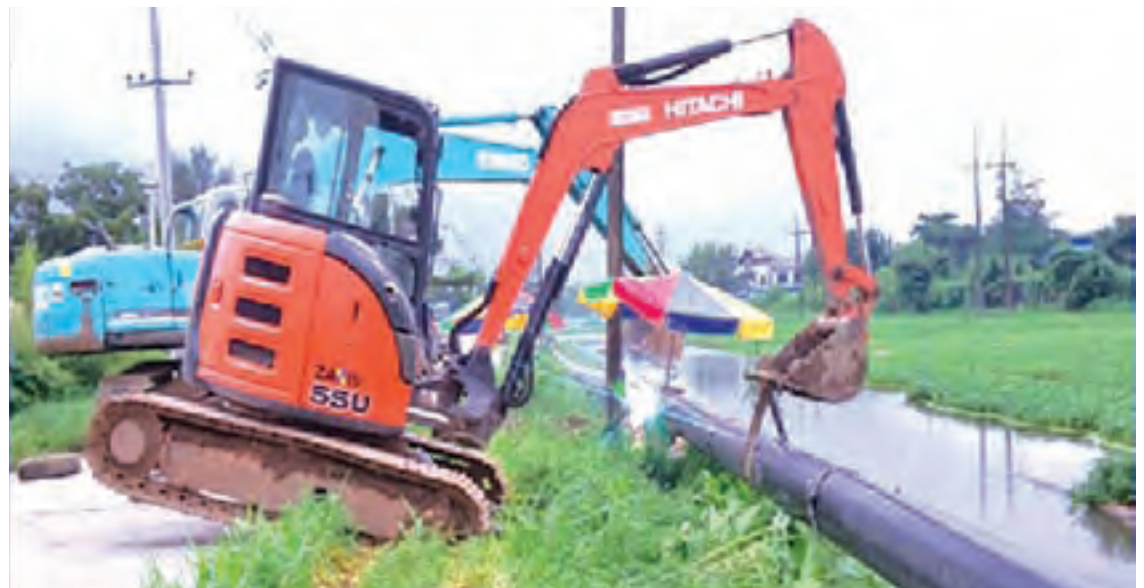
Fixing and replacing of natural gas pipelines along the Yangon and Mandalay Region.
