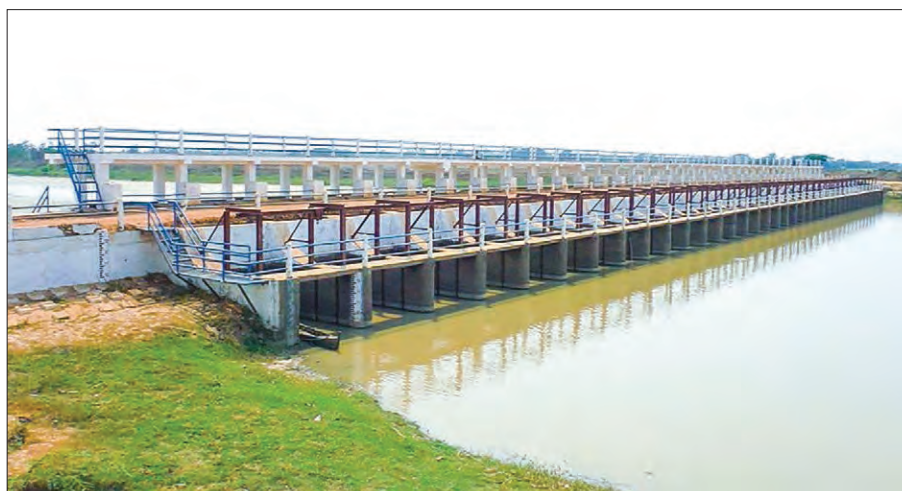
Paing Kyone sluice gate that regulate sewage in the river. PHOTO: MNA
