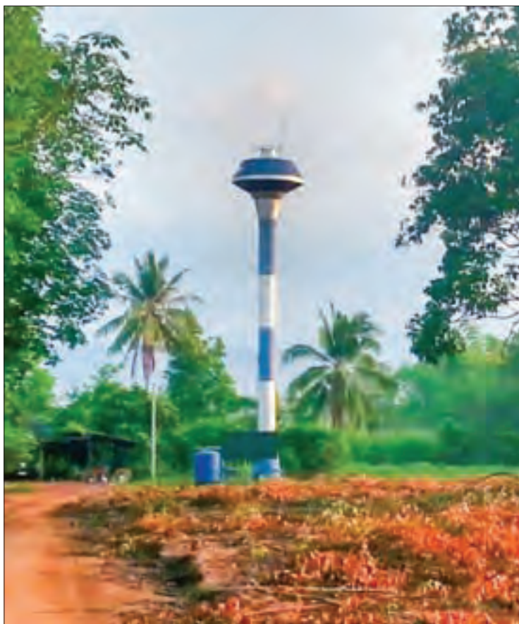
Village water supply system in rural Thailand.
