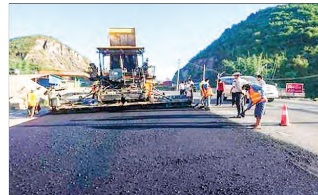
Mandalay-Lashio Road is being expanded. PHOTO: MNA
