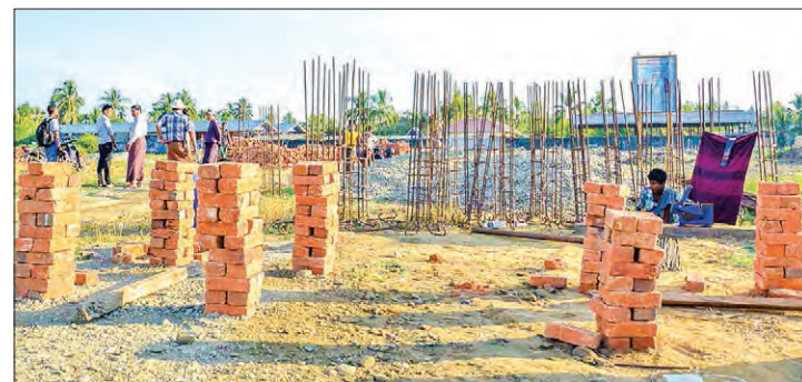
The construction of indoor stadium in Maungtaw. PHOTO: THIHA SITHU
