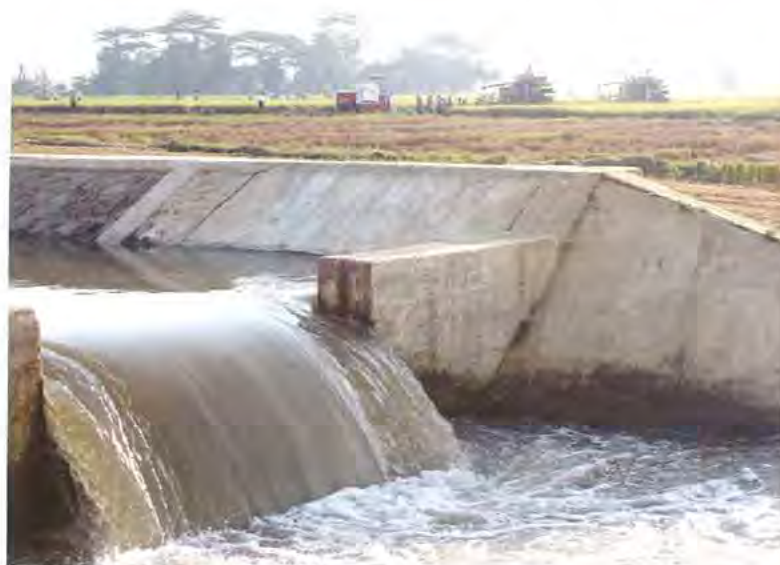
Constructed River Water Pumping Projects
