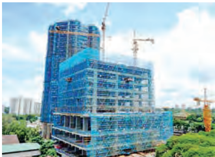
Kanthaya Consortium Towers being seen under construction.
