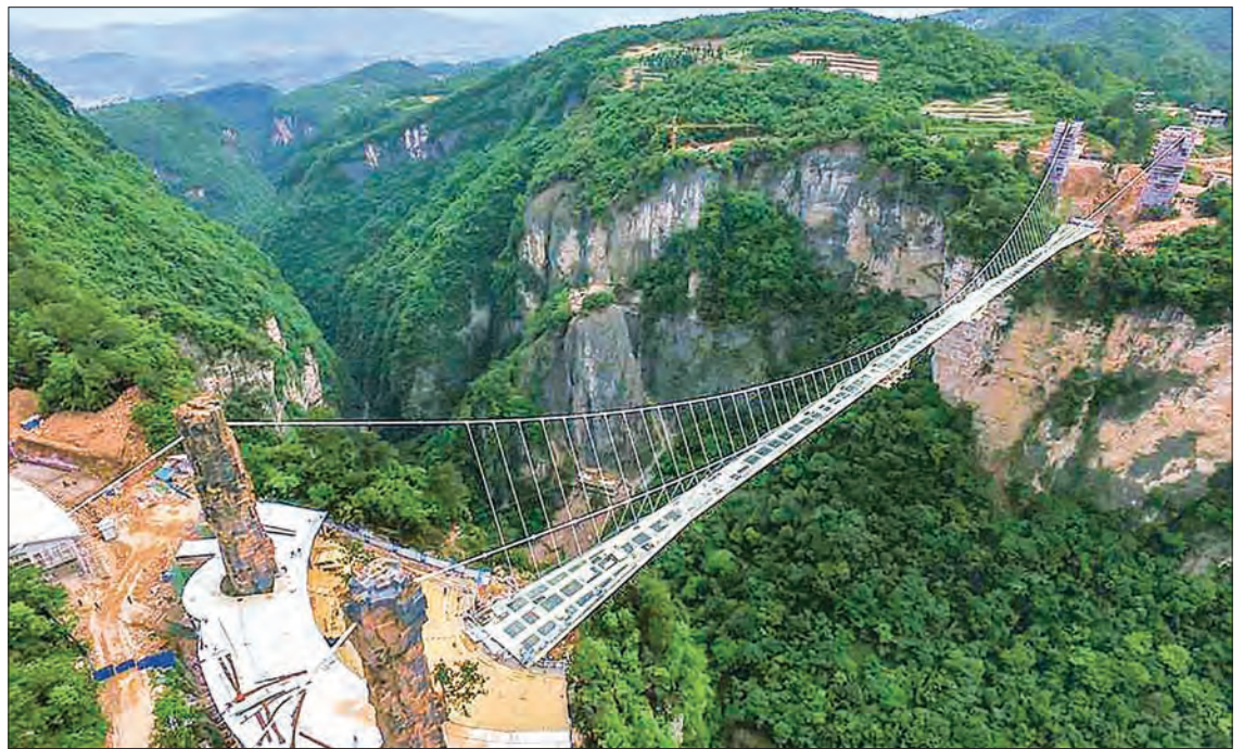
An aerial photo taken on 17 May, 2016 shows the construction site of a glass bridge at the Grand Canyon of Zhangjiajie National Forest Park, central China's Hunan Province. The 430-metre-long, 6-metre-wide bridge is expected to be put into a trial operation in May. The structure has undergone nearly 100 safety tests to ensure that it can support the weight of 800 people. PHOTO: XINHUA
