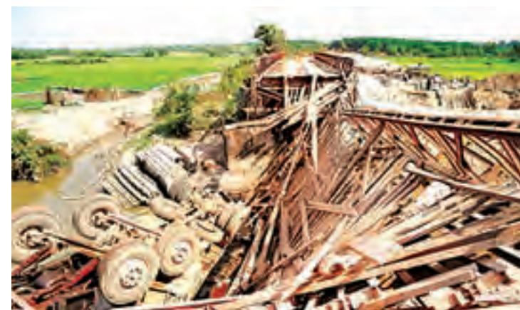
Bridge collapses due to an overloaded truck. PHOTO: NAING TUN (IPRD)
